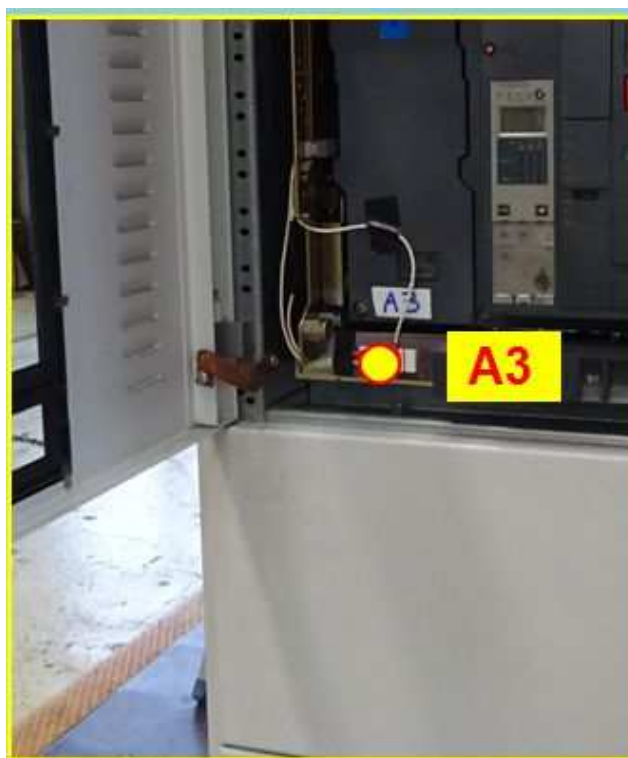
Photo 5: A3 Measuring point placed on the switchgear support
